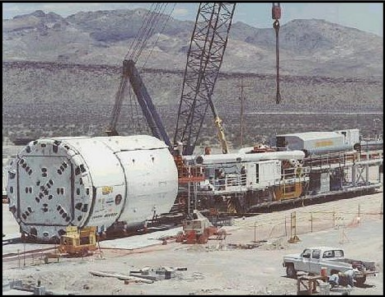
Tunnel Boring Machine (TBM) used to excavate the ESF.
