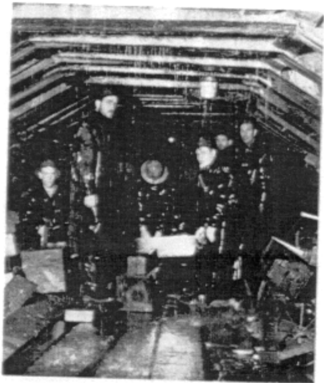
Ever-present seepage was only one obstacle to completing San Jacinto Tunnel.
